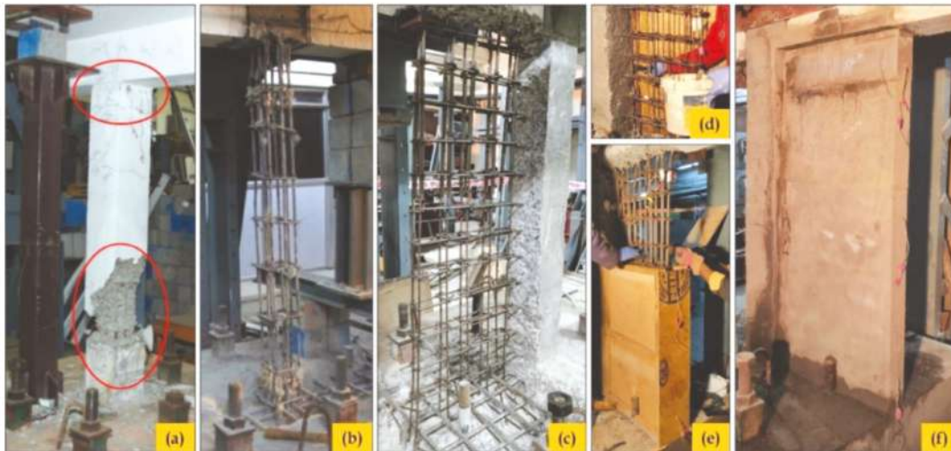
Sequence of retrofitting of the damaged ground story columns using shear walls
